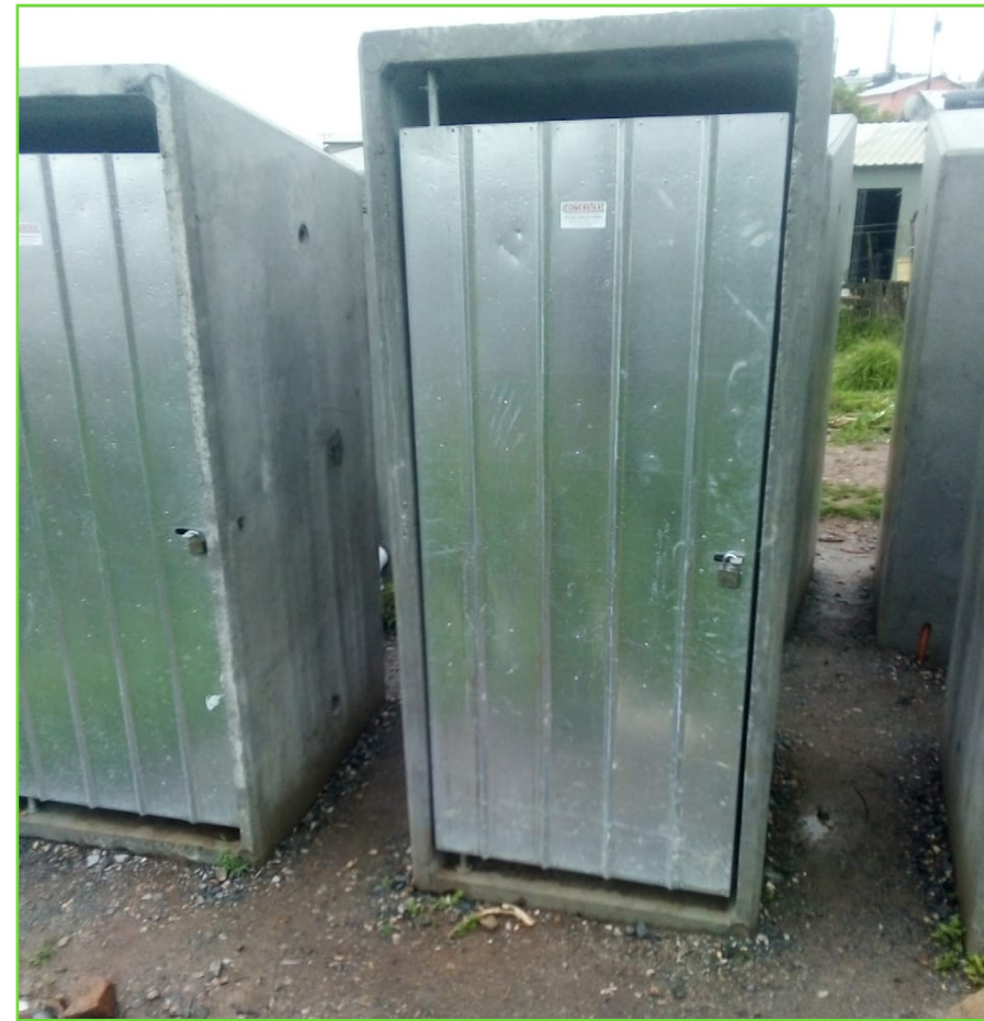
Newly installed toilets at Bossiesgif, Bitou
